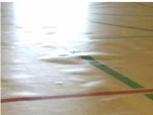
Picture above: Damaged floor coatings due to moisture vapor issues
